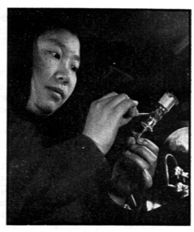
Components are assembled as above where capacitors and vacuum tubes receive the dextrous attention of Chinese employees. Below, a worker finishes up the wiring on a transmitter, while a coolie, right, forms the local version of a conveyor line in transporting units around the plant
